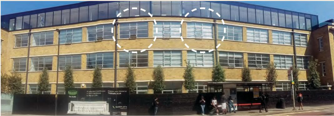
London office building converted to apartments. Fitted with new double glazing with a U-value of 1.1
